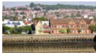
Aveling & Porter building immediately before demolition in 2010
