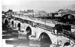
The old bridge to be demolished and new Rochester Bridge in background
